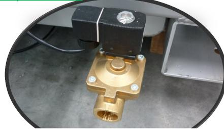
The water fill valve turns on to fill the sump when the ambient temperature reaches about 70 degrees
